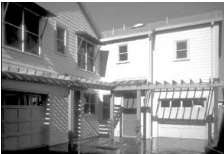
Awning and Trellises to Reduce Heat Gain
