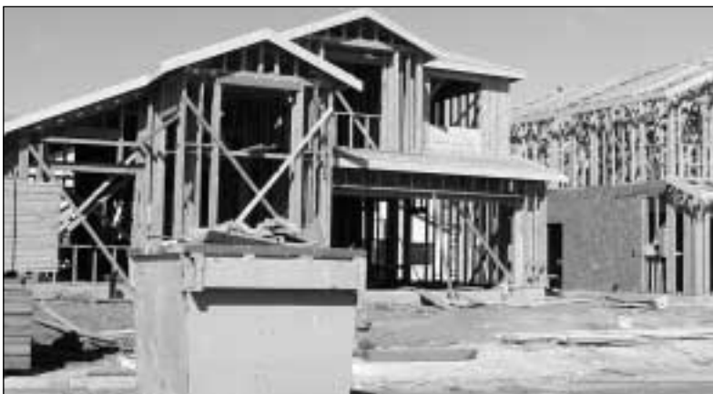
Job Site Recycling, Foothill Glen Housing, Union City, CA
