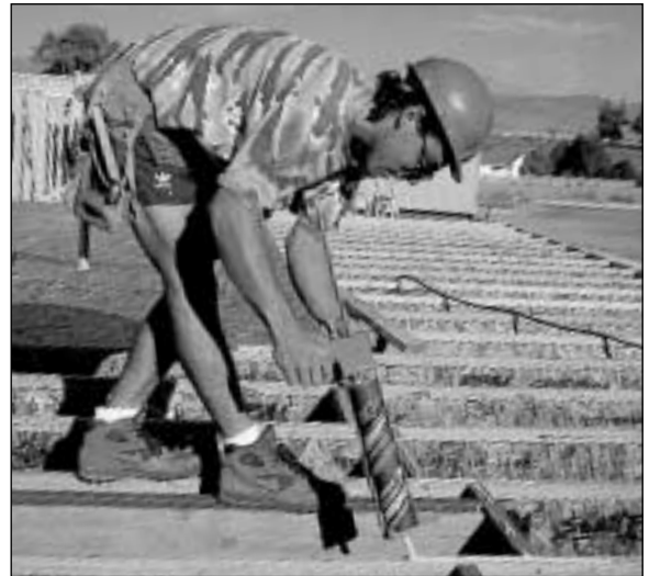
Using Solvent-Free Adhesives
