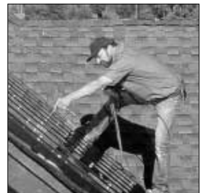
Installing Solar Water System
