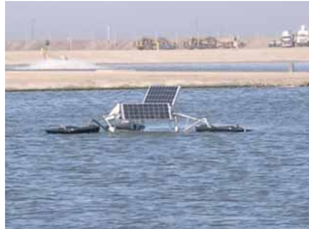
FIGURE 6 SOLAR-POWERED AERATOR/MIXER (COURTESY SOLARBEE)
