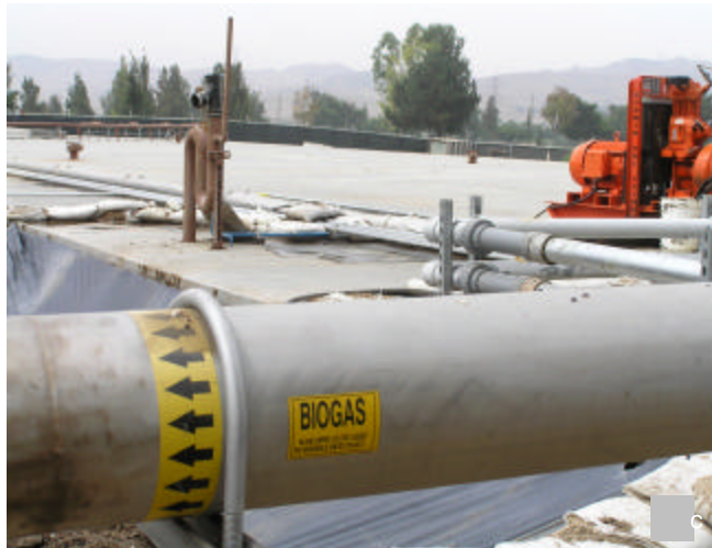
Figure 13. IEUA cogen desalting plant. Manure generated on dairies (a) is transported to digester (b & c) where power is produced to operate a groundwater desalting plant (d).
