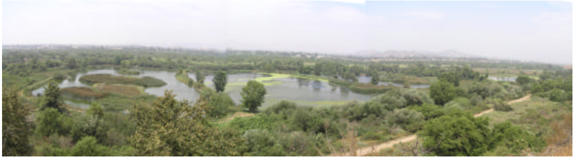
Figure 18. The City of Riverside constructed this 14 mgd wetland to remove nitrogen prior to discharge to the Santa Ana River.
