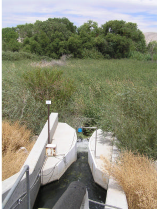
Figure 8. City of Victorville's outfall weir into the Mojave River
