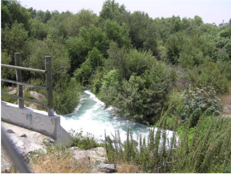
Figure 16. City of Riverside's 30 mgd flow leaving the treatment plant via a discharge channel connecting to the Santa Ana River
