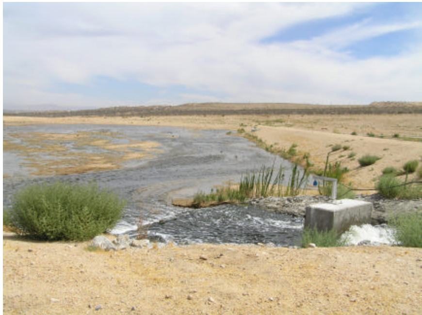
Figure 9. One of Victorville's infiltration basins adjacent to Mojave River
