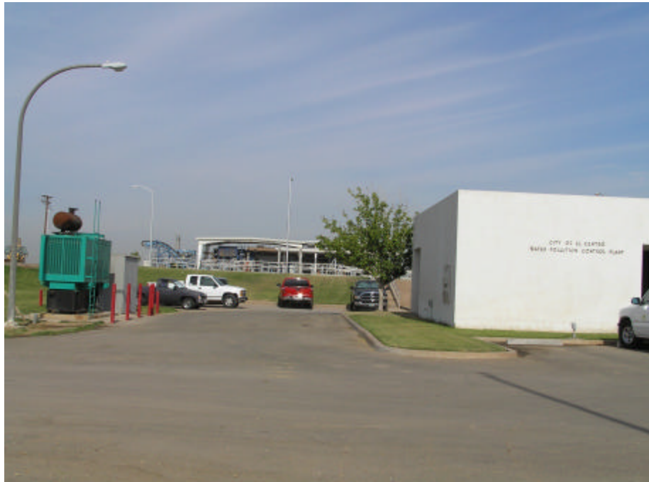
Figure 10. City of El Centro treatment plant
