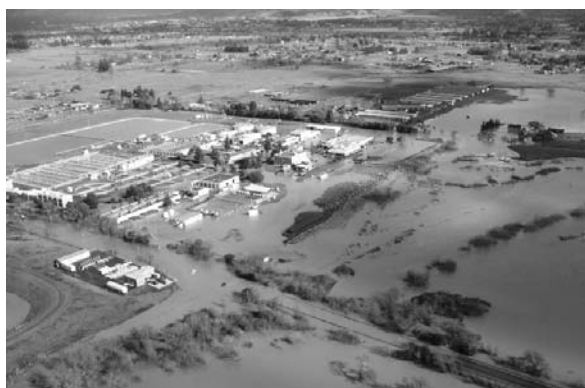
Winter storms led to unprecedented flooding at the Laguna Wastewater Treatment Plant.
