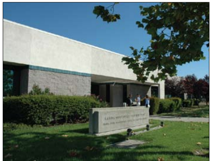
Headquarters for the Laguna Wastewater Treatment Plant.
