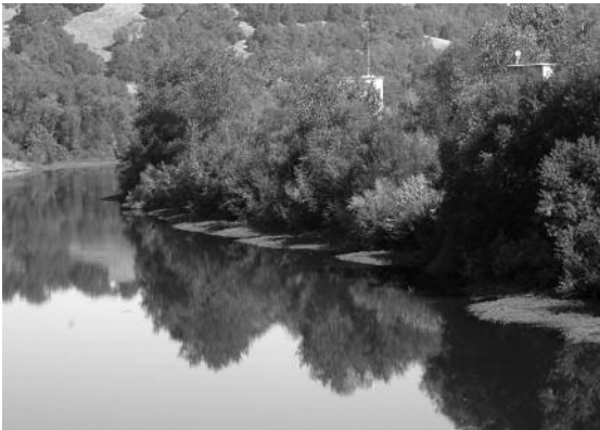
Water intakes on the Russian River near Wohler Bridge.
