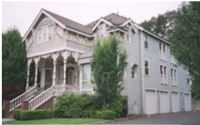
A reconstructed building in the St. Rose Preservation District retains the original façade elements while new construction to the rear provides units in the downtown area.
