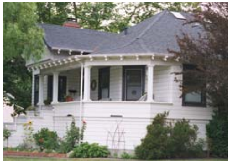
A porch is one of the main defining features of a house and should not be enclosed or removed.
