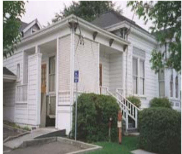
Mechanical lift is screened by lattice work on this Queen Anne house used as an office.
