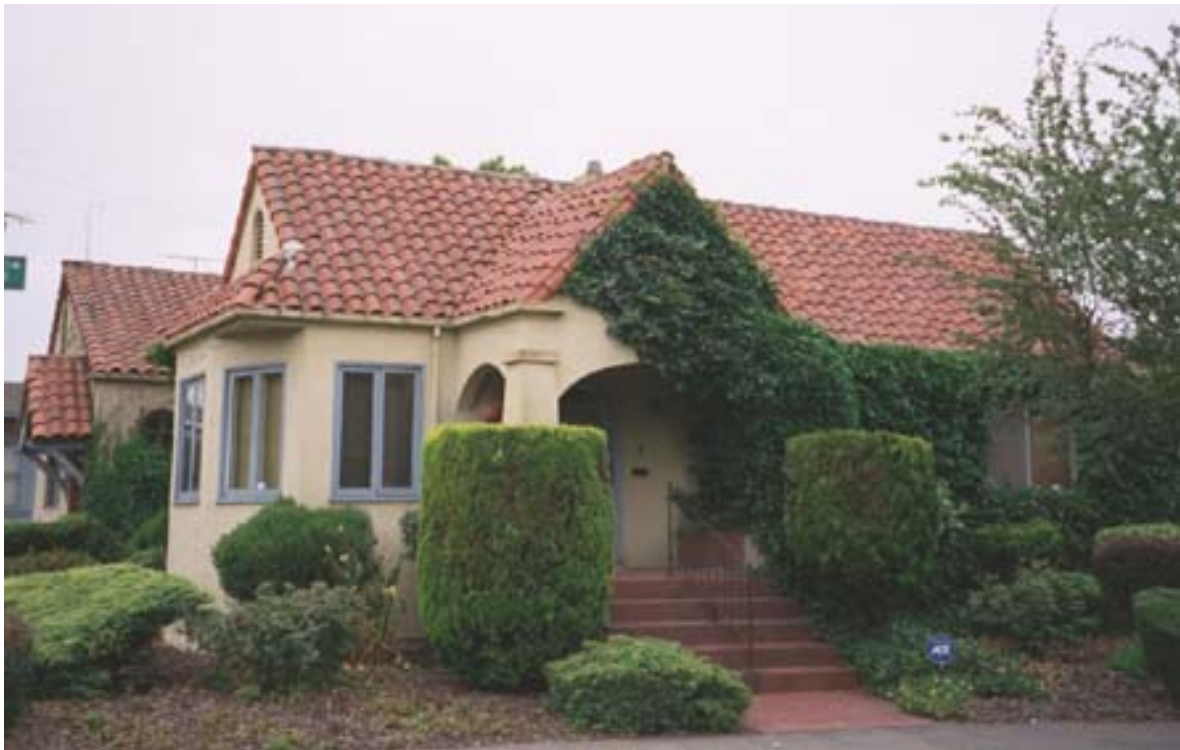
Tile roofing is an integral part of this Mediterranean Revival house's character.
