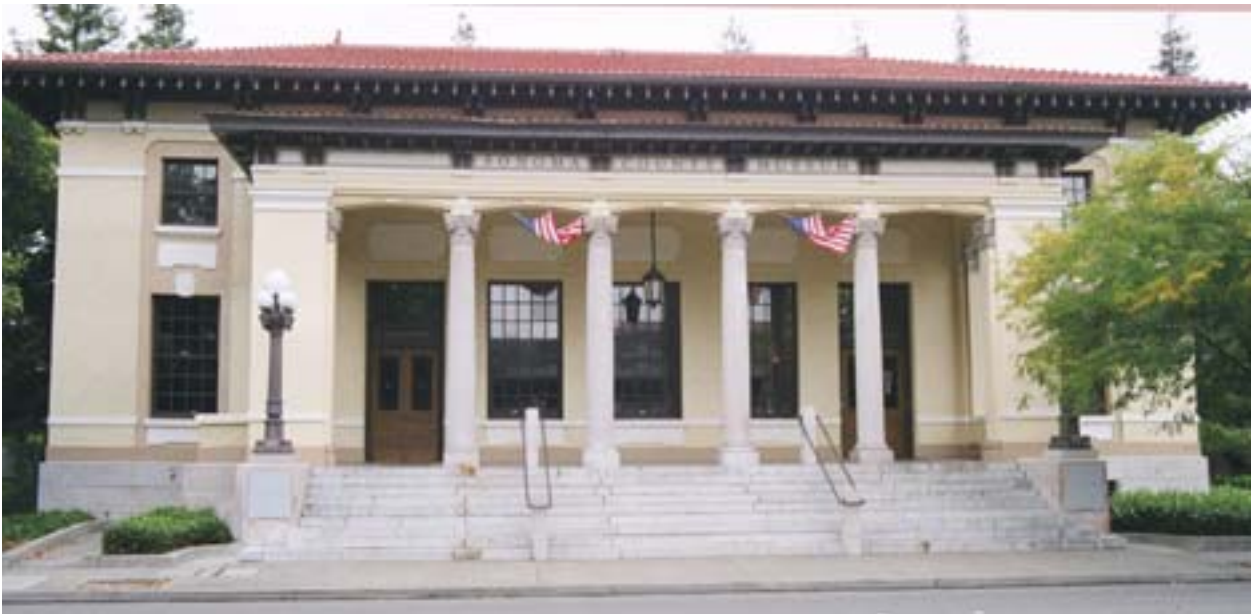
The old Santa Rosa Post Office, a Roman Renaissance Style building, was moved from its Fifth Street site (in a Redevelopment area) to its current Seventh Street location in the St. Rose Preservation District. The restored landmark houses the Sonoma County Museum.
