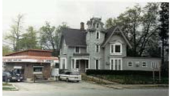
Insensitive new construction, along with an inappropriate addition, has compromised the integrity of this Gothic Revival Style house.
