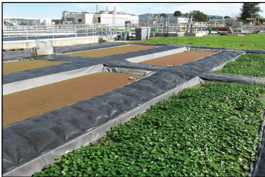
Channelized Wetlands at the Laguna Treatment Plant
