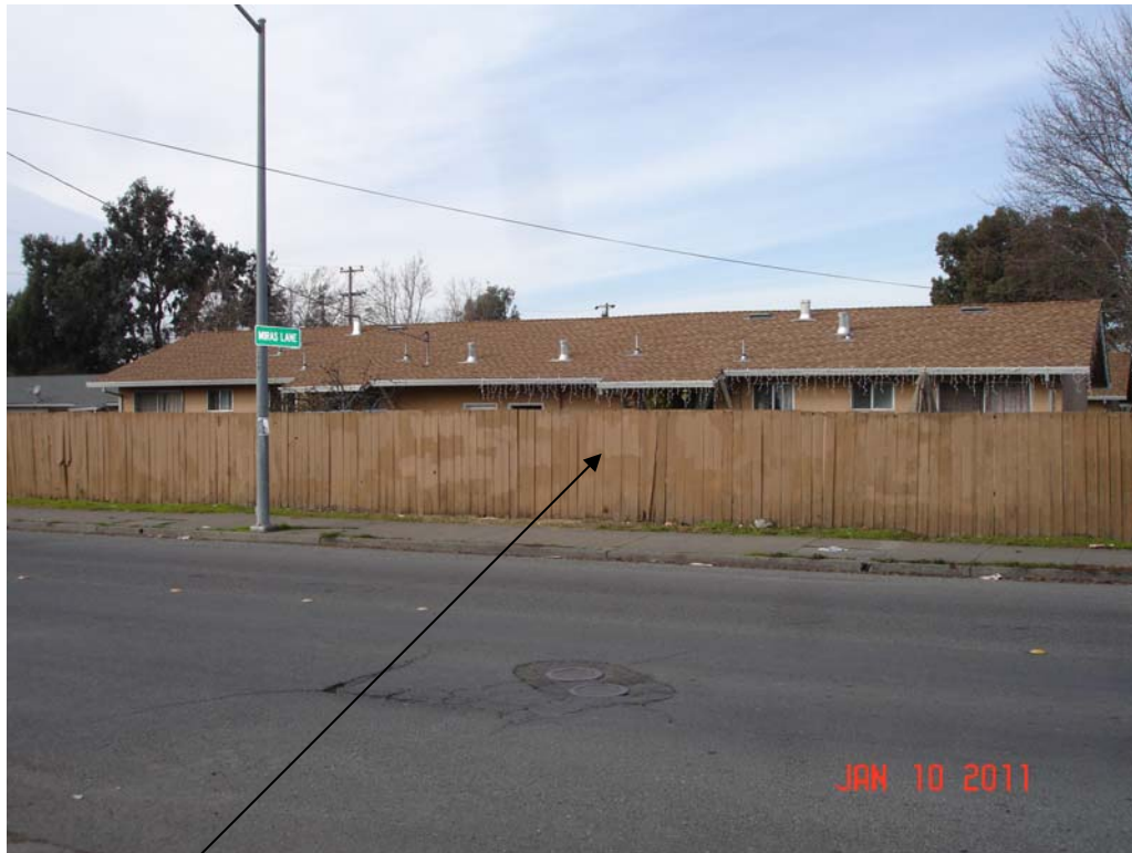
Main fence facing Aston Ave (approx. 86'4")
