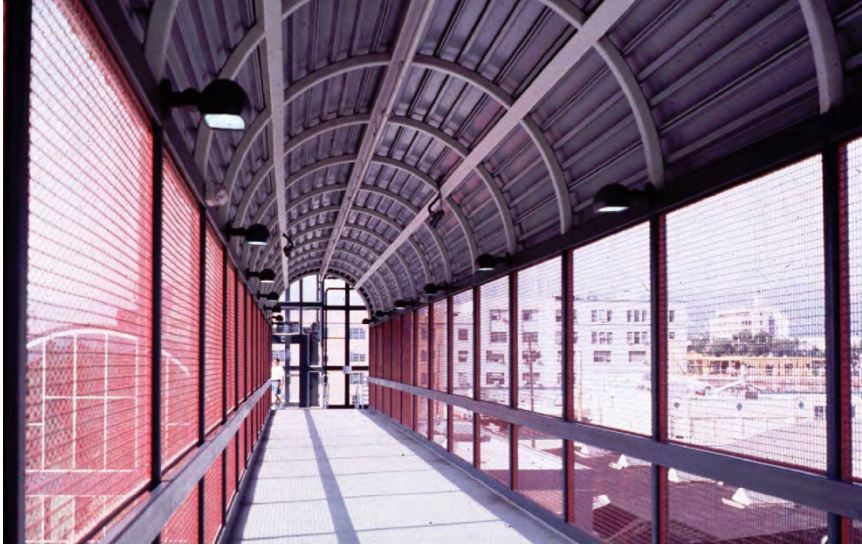
Figure 3.4 Fencing on Pedestrian Bridge at Jack London Square, Oakland retains its transparency for people crossing the tracks.
