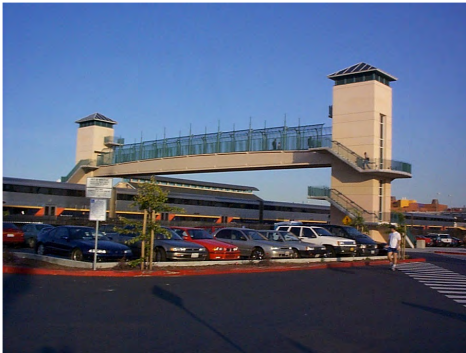
Figure 3.3 Fencing on both the Jack London Square/Oakland Amtrak Station Bridge (top) and the Emeryville Amtrak Station Bridge (above) show high transparency when viewed from a distance.
